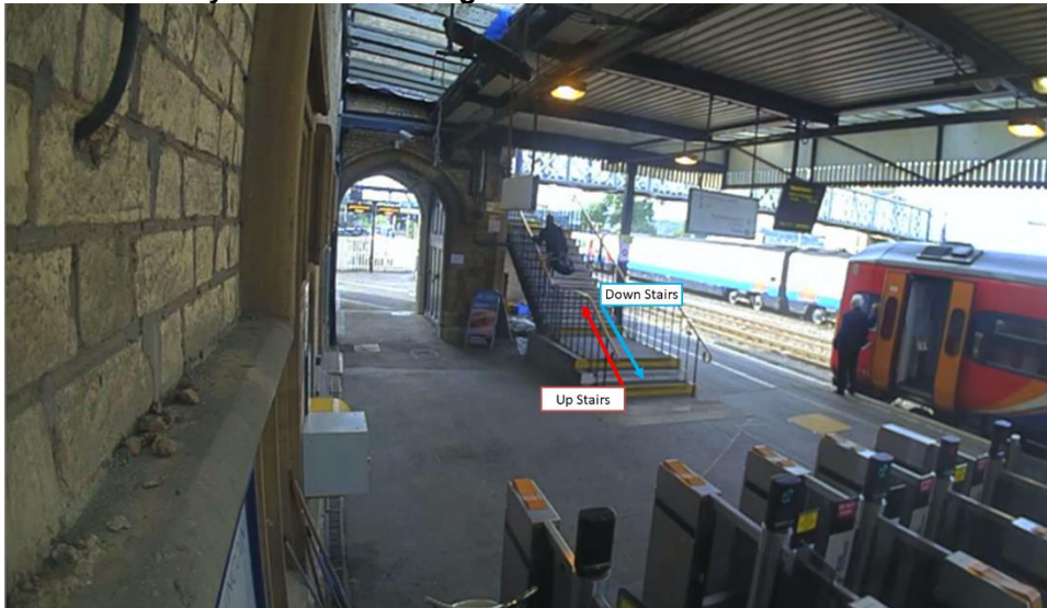
Public Footbridge over Railway
